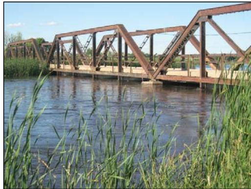
This is an historical truss bridge near Lewellyn. Engineers had to cut channels on both sides through the road to save the bridge. The road has not been repaired yet so the people who live on the south side have to drive a few miles on east to Highway 26 and the new bridge.
